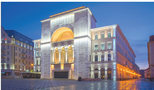
Romanian Opera House, (Piața Operei)
