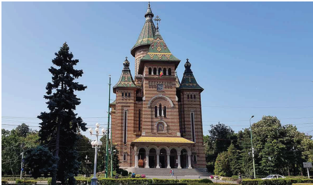
Timișoara Metropolitan Cathedral, Bulevardul Regele Ferdinand I, Timișoara, Romania
